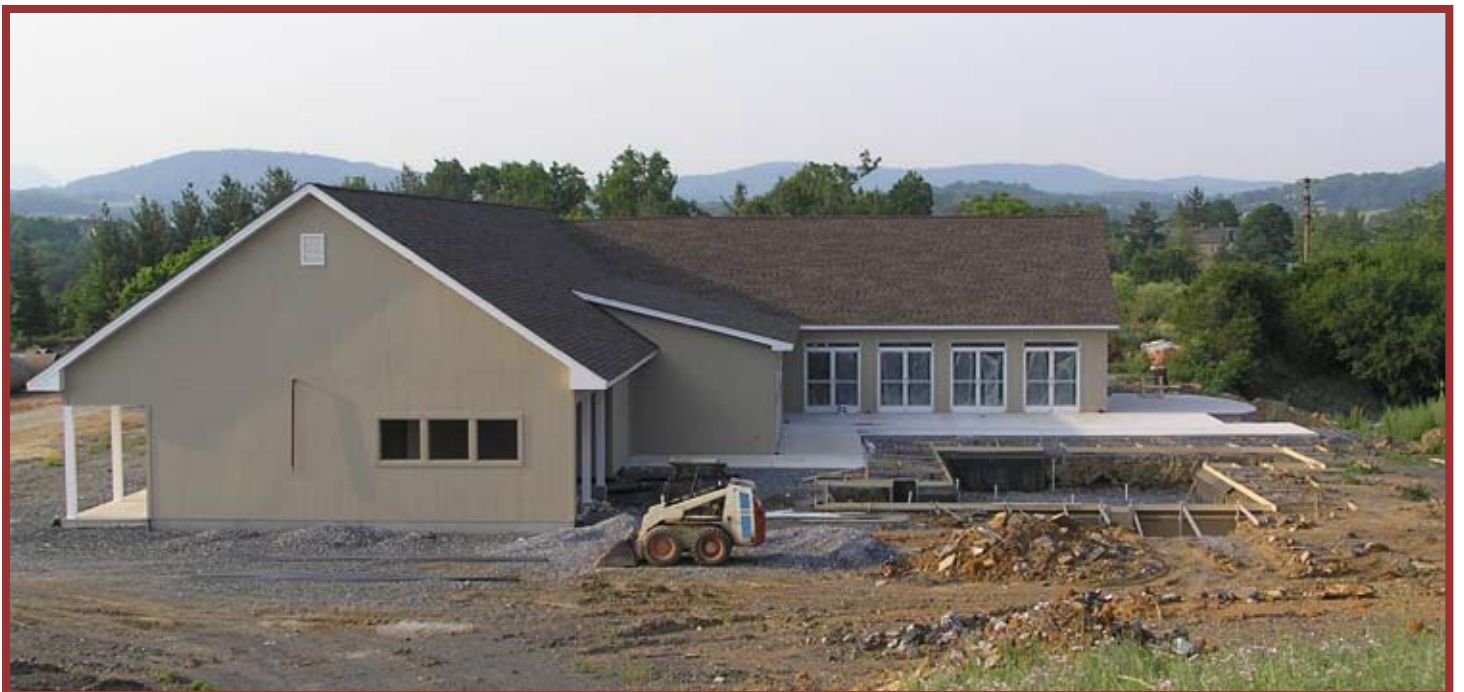
Recreation Center outdoor recreational pool and sundeck under construction.
